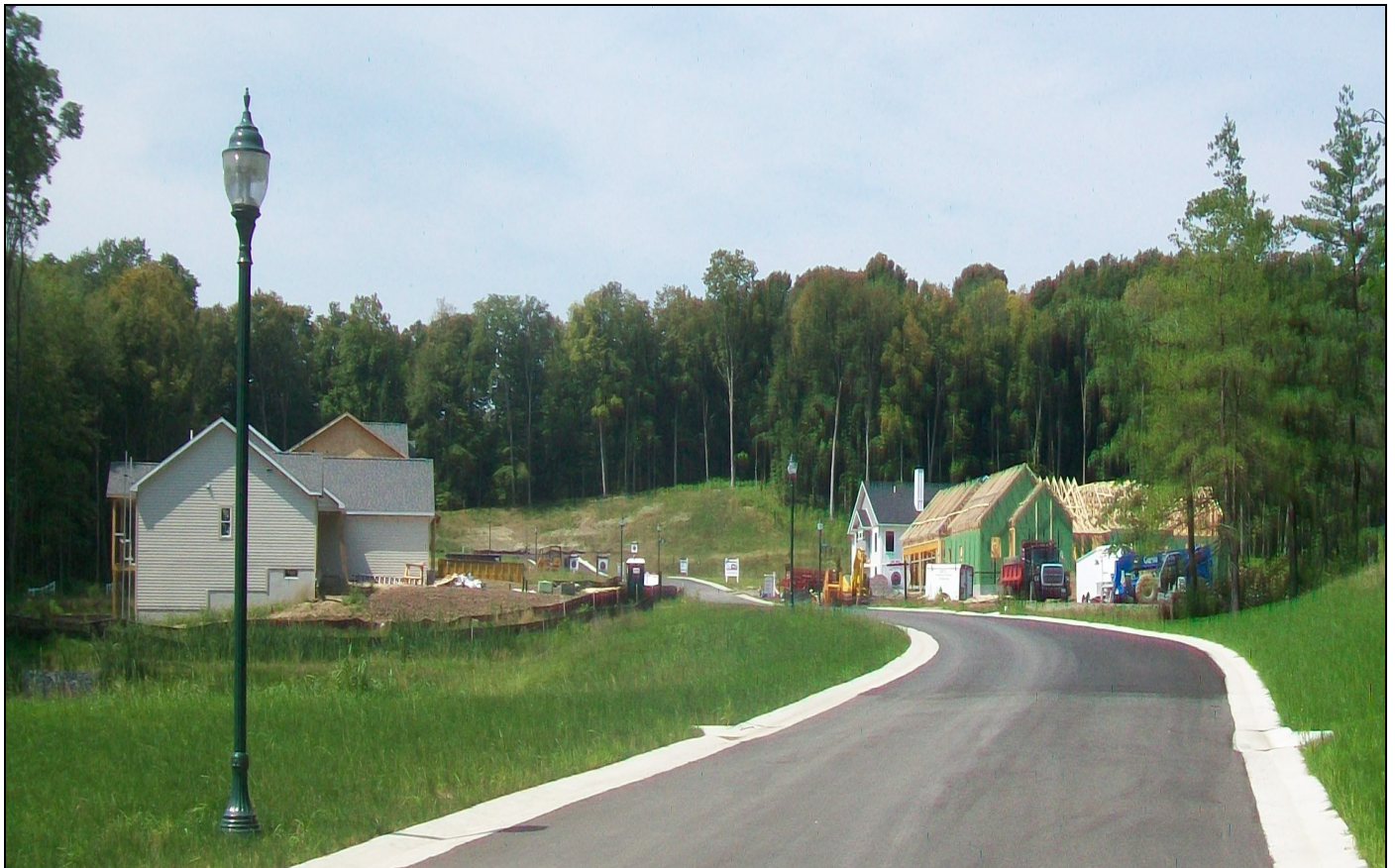
Progress at Baltimore Ridge
