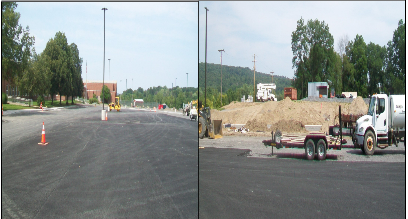
Construction at Marcellus High School
